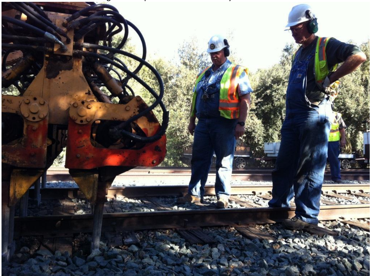
Chris and Steve judge the effort of the tamper in stabling the area at MP 1.85
