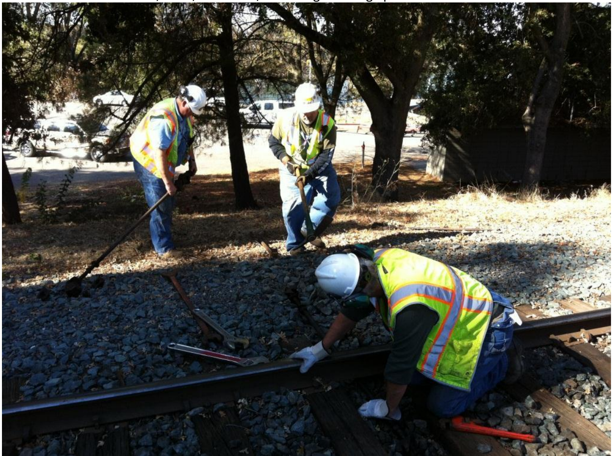
Chris adjusting a gauge-rod as Mike digs under the rod that Steve is installing
