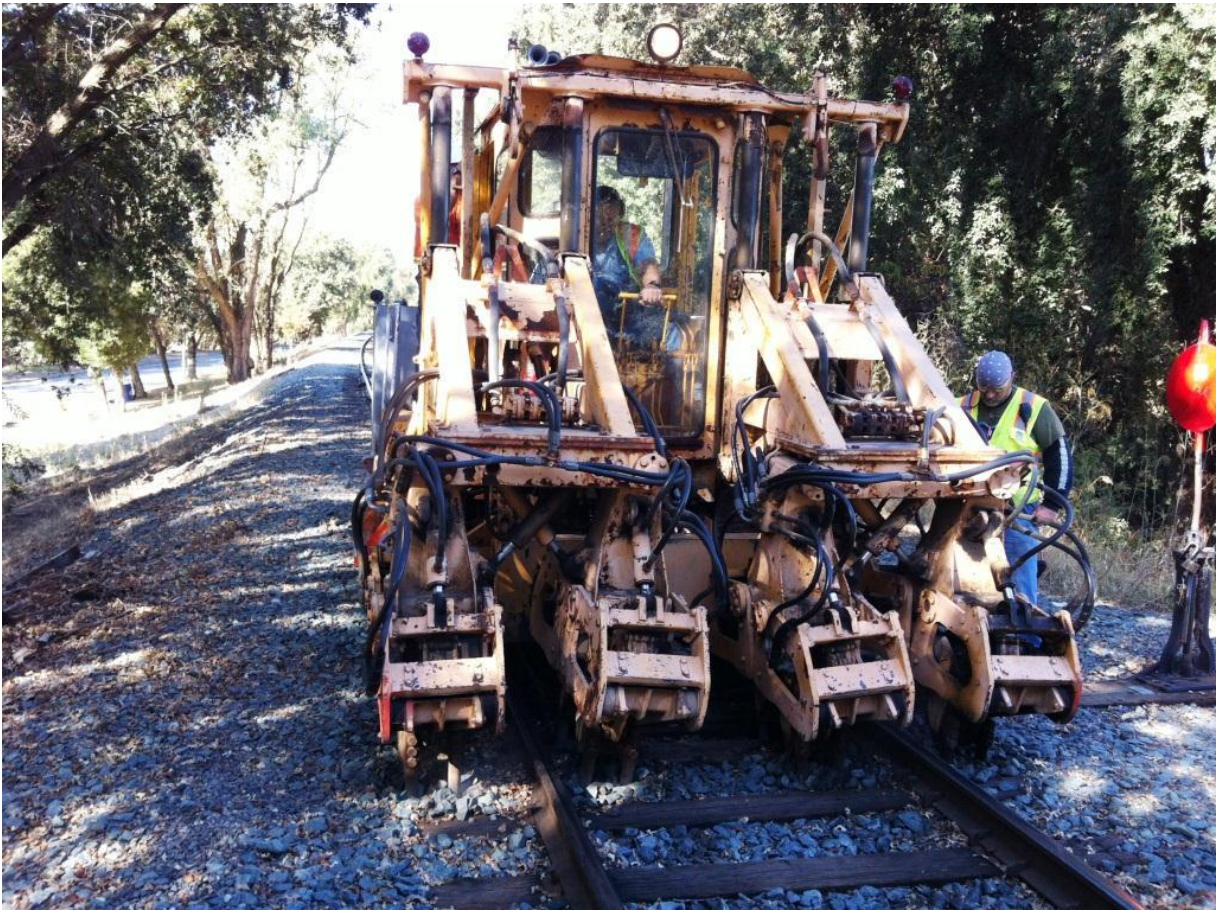
Chris controlling the tramper while Mike manually activates that actuators
