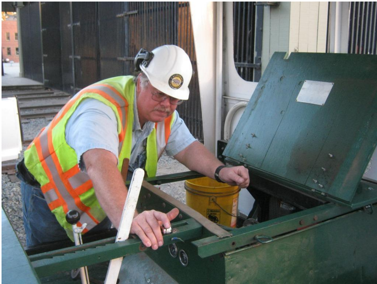
Chris making repairs to the MW 51 Motorcar
